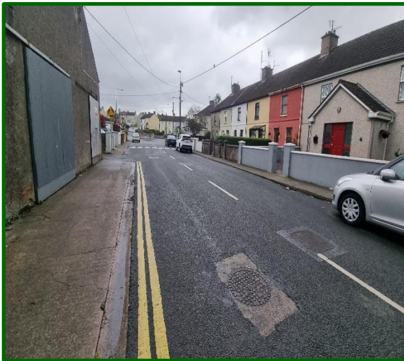
Picture 4: Photograph showing road on-site
