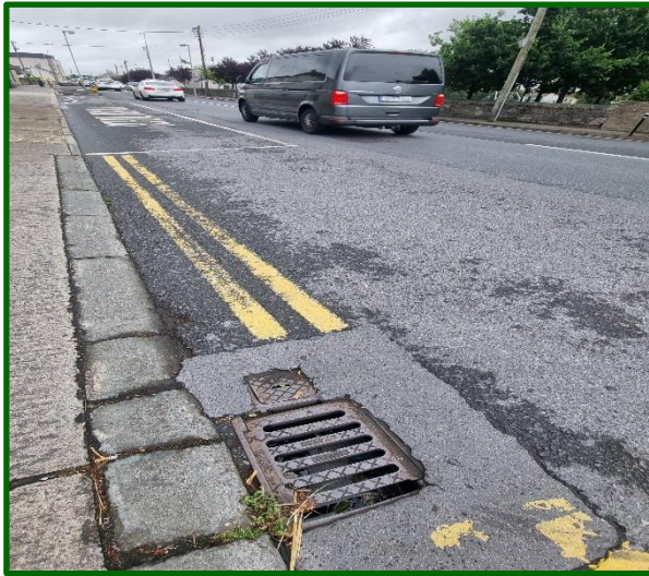
Picture 1: Photograph showing surface water drains on site
