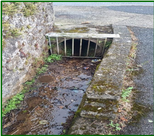
Picture 1: Photograph showing storm drain on-site
