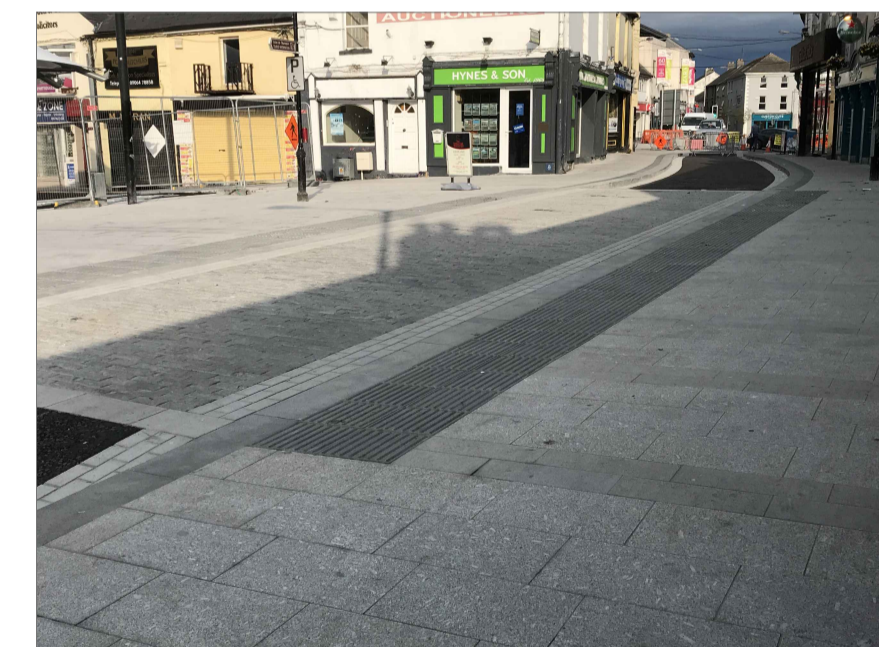
Kerbs - Flush and Raised - Irish Limestone
