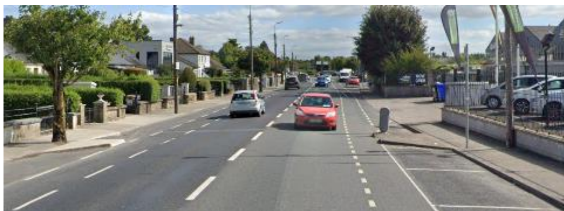
Figure 6-4: Space available on Davis Road
