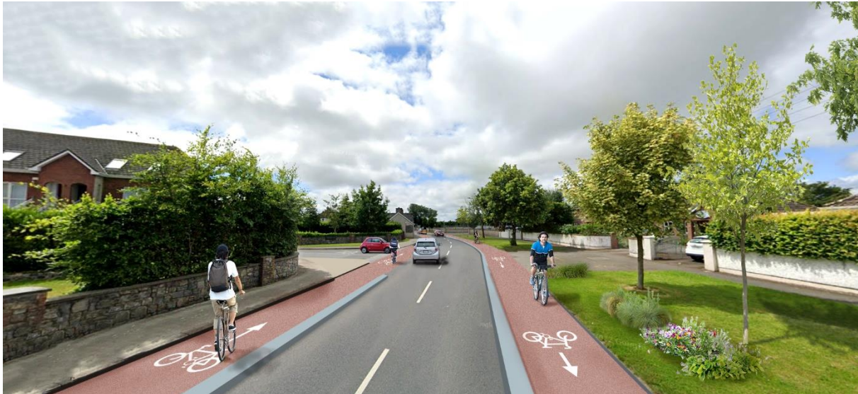
Figure 6.5: Example of Segregated Cycle Route along R659, north of Co-Op Livestock Mart
