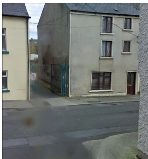
Figure 6-11: Gordon Place Car Park Access
