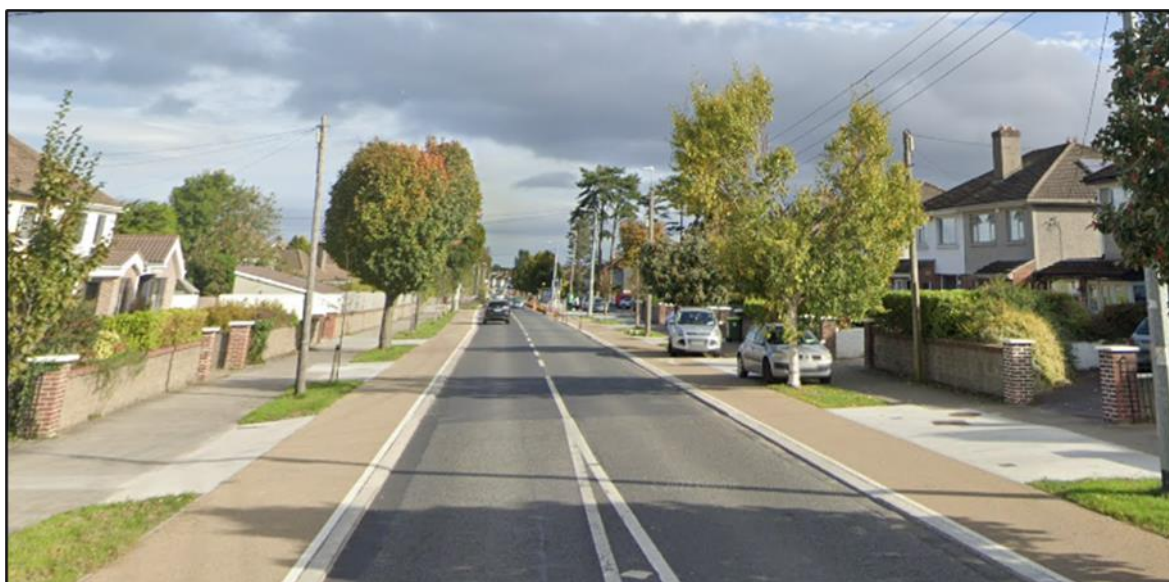
Figure 4-2: Example of a Segregated Cycle Track
