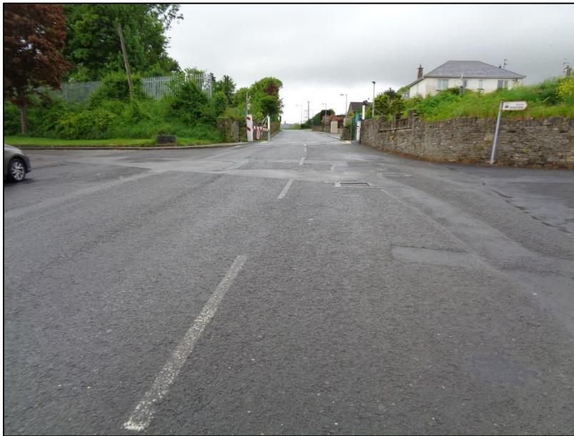
Pl. 5. Looking North at Cregg Road/Marian Avenue/ Railway Station Road Junction.
