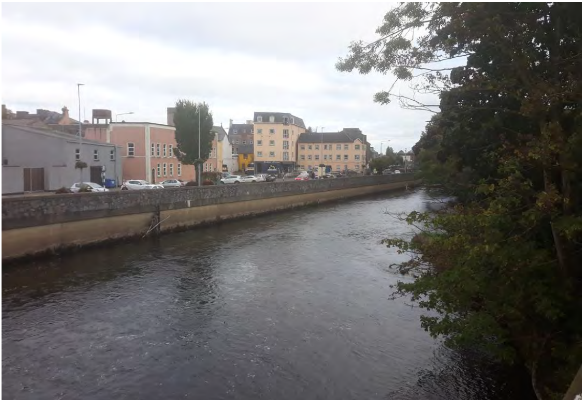
Photo 3: View of North Plaza from Old Bridge walkway looking downstream
