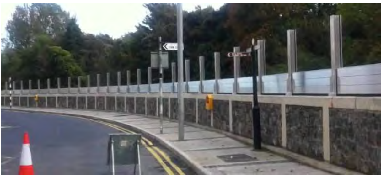
Figure 1: Demountable barrier system
