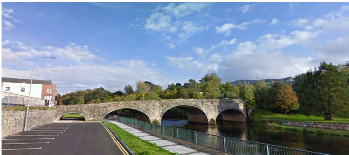
Photo 11: Old Waterford Gashouse Bridge looking in downstream direction
