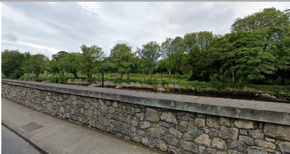
Photo 10: Bridge 2 crossing looking from Raheen Road to Suir Island
