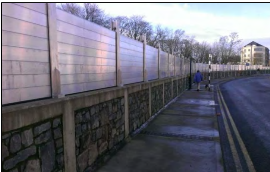
Figure 3-10: The Quays demountable barrier system
