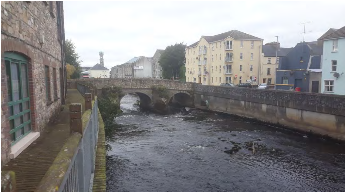
Photo 9: View of Old Bridge Road northern river reach crossing looking upstream
