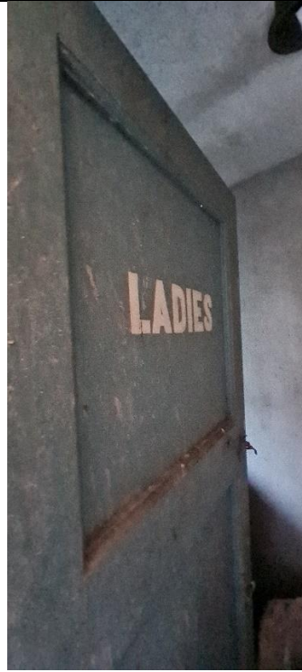
A10: Entrance to ladies' toilet off south-east external passage
