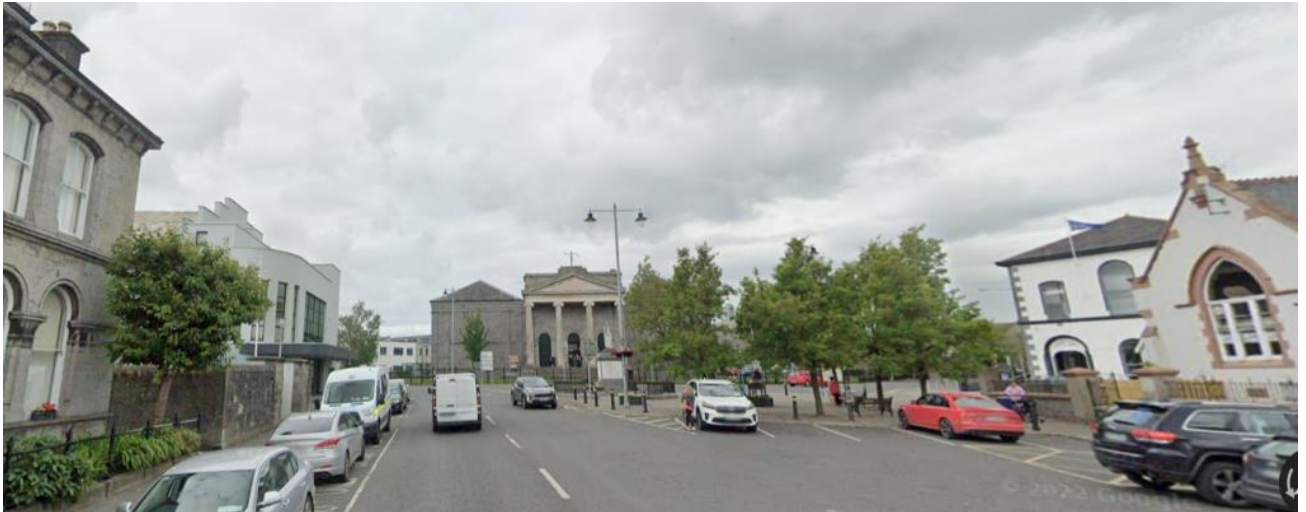
Fig. 5 Recent photograph of Banba Square looking north-west towards the courthouse (centre, with republican memorial in front) with the former bank (now Garda Station, foreground) and the vacant Rialto Cinema (background) on the left, and the former Presbyterian Church (now tourism information office, foreground) and town hall (now Nenagh Arts Centre, background) on the right.
