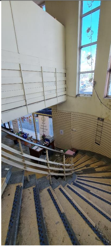
A22: Curved staircase & first floor landing
