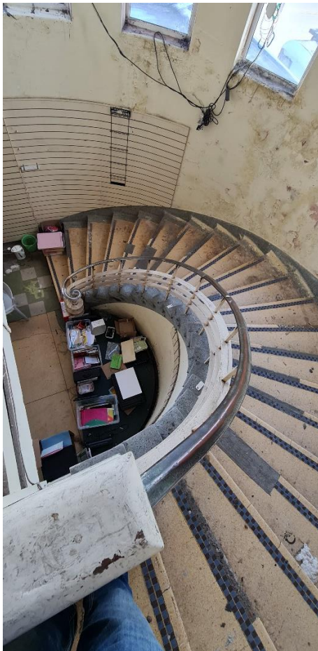
Fig. 19 Curved staircase to first floor foyer – to be retained
