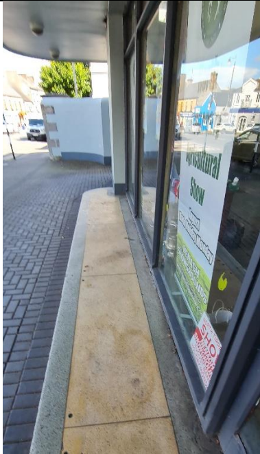
A5: Terrazzo Step at entrance to former cinema
