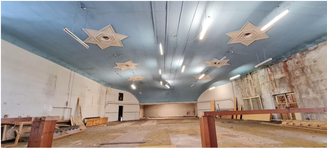
Fig. 13 The curved plaster ceiling, with art deco details, survives in an intact condition above the later (post-1976) mezzanine floor.
