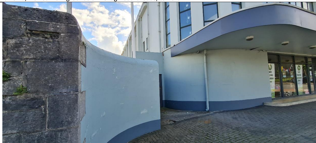
A3: East corner of former Rialto Cinema – the curved boundary wall of Nenagh Garda Station (formerly the Provincial Bank) echoes the curve of the cantilevered canopy and external wall of the main staircase
