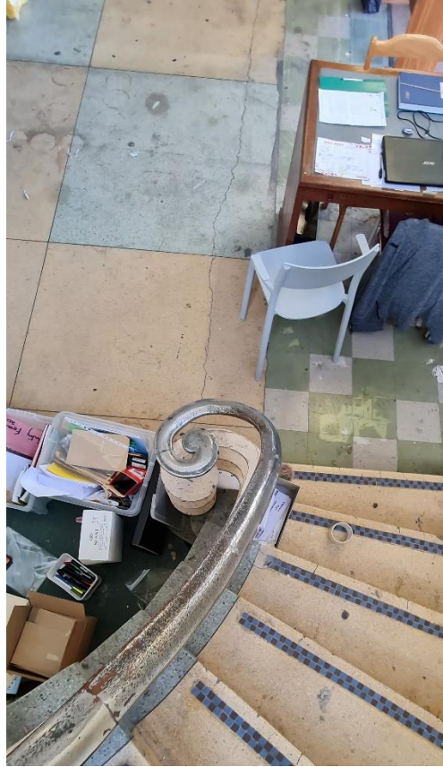
A19: Curved staircase
