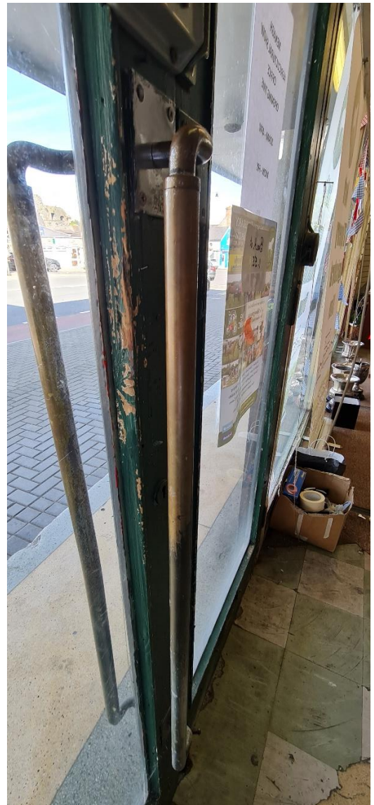
Fig. 23 Curved brass pull handles on timber double doors at entrance to former Rialto Cinema
