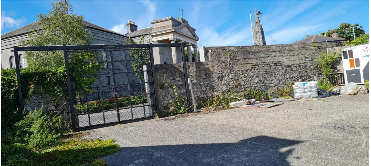
Fig. 25 Stone rubble boundary wall to north of cinema, with gate onto Ashe Road. The portico of Nenagh Courthouse is visible in the background.
