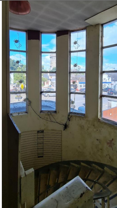
A23: Curved external wall of main staircase
