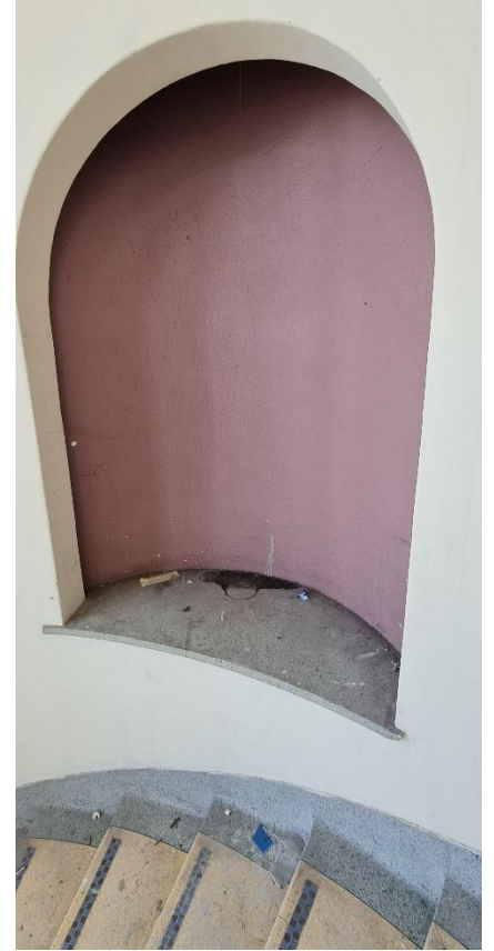
A20: Niche off curved staircase
