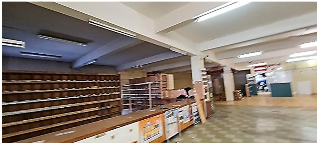
Fig. 15 Ground floor photograph showing post-1976 mezzanine floor to be removed and replaced. The inclusion of an open stairwell within the centre of the space will create an important visual connection between the two levels of the former auditorium.
