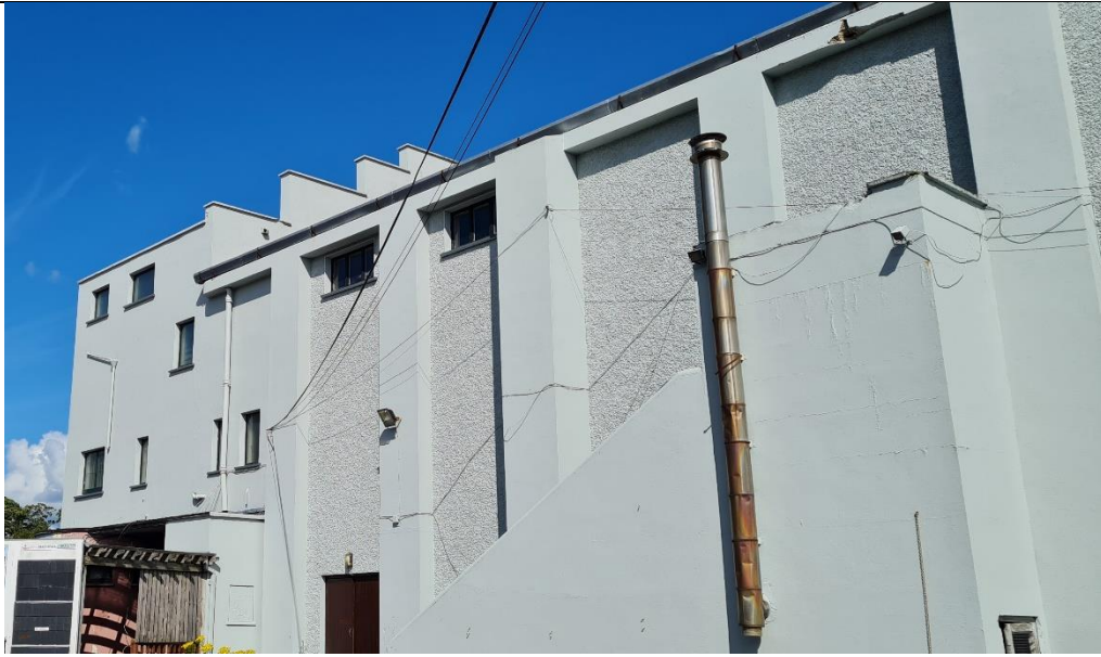
A8: Detail of north-west (side) façade of former Rialto Cinema
