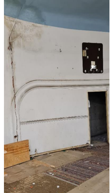
A28: Decorative plaster detail on chamfered wall on left of former cinema screen
