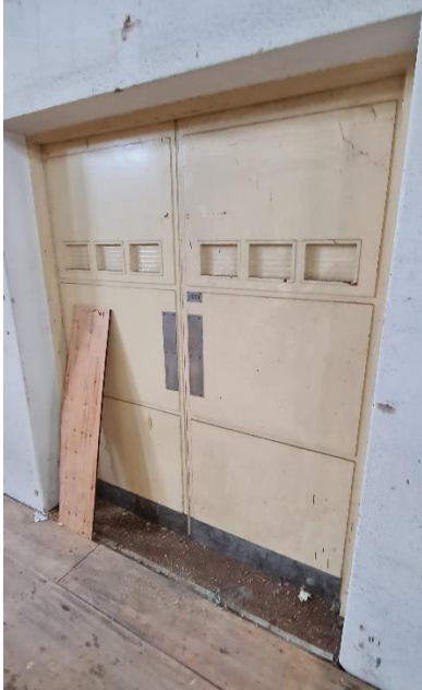
A26: Double doors from former gallery to first floor landing
