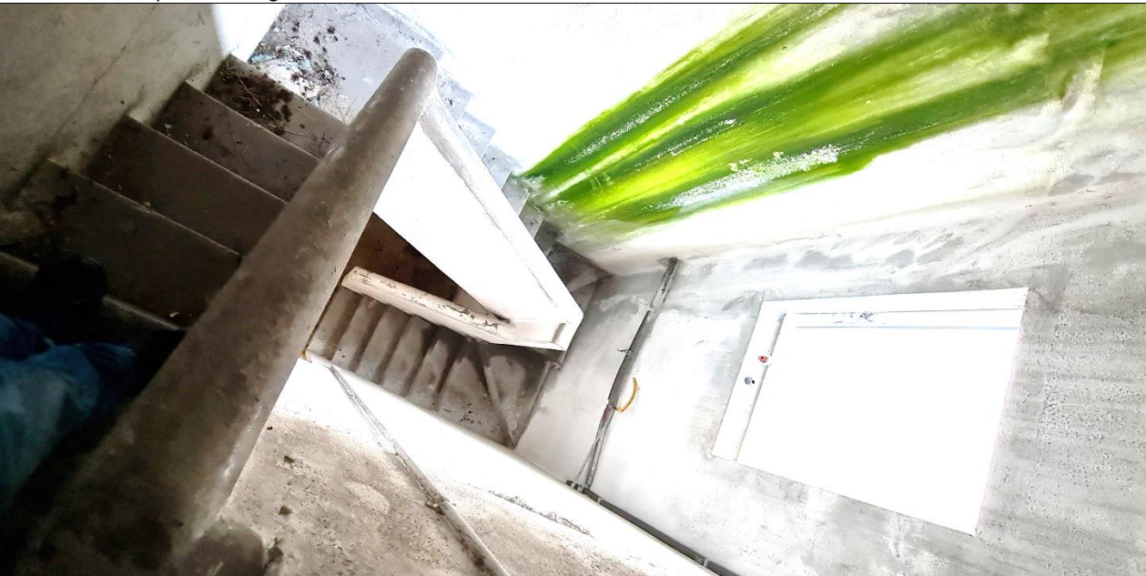
A30: Service staircase from first floor (public landing) to projection booth
