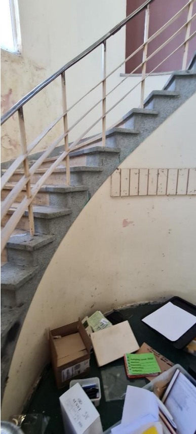
A18: Curved staircase
