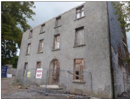
Plate 9 Suir Island House façade (note the slate on the side elevation (southern) and return) Plate 10 Side elevation of the return building
