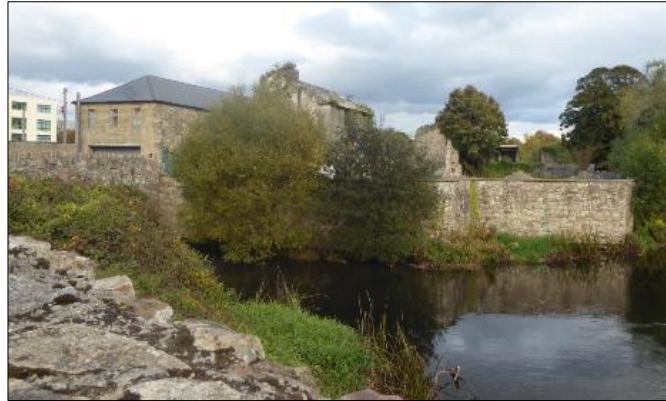
Plate 3 New flood defence walls on the south westernmost end of Suir Island-Willow Island
