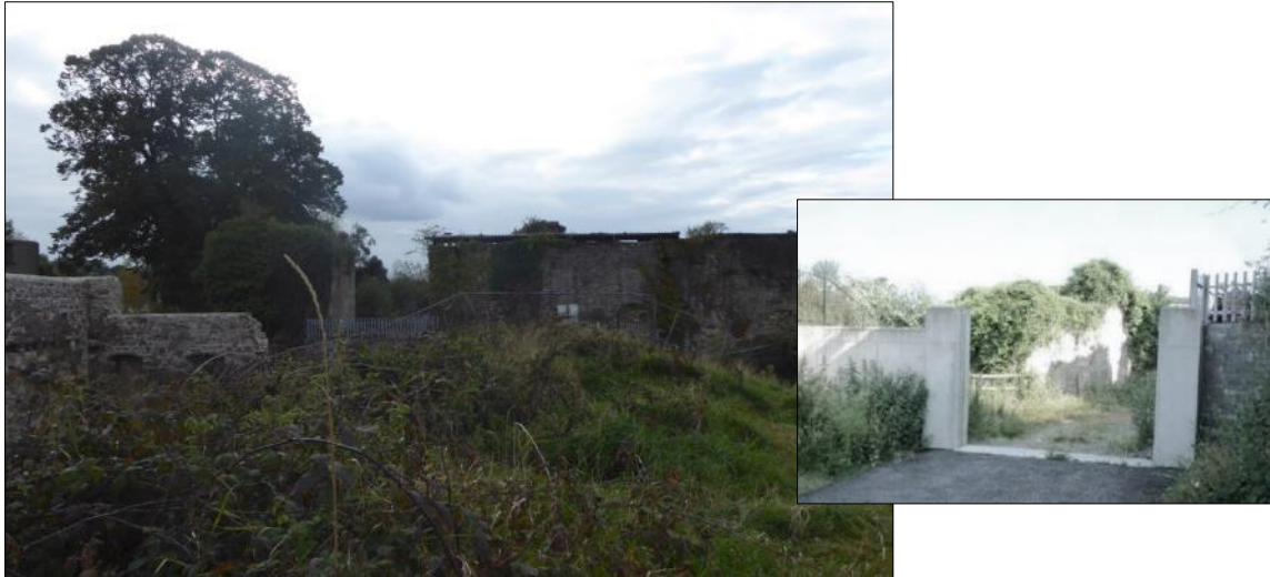
Plate 6 View looking west (from ontop of the berm in the car park) showing the ‘tower’ over grown in ivy and the roofless stores building, (inset: the entrance)
