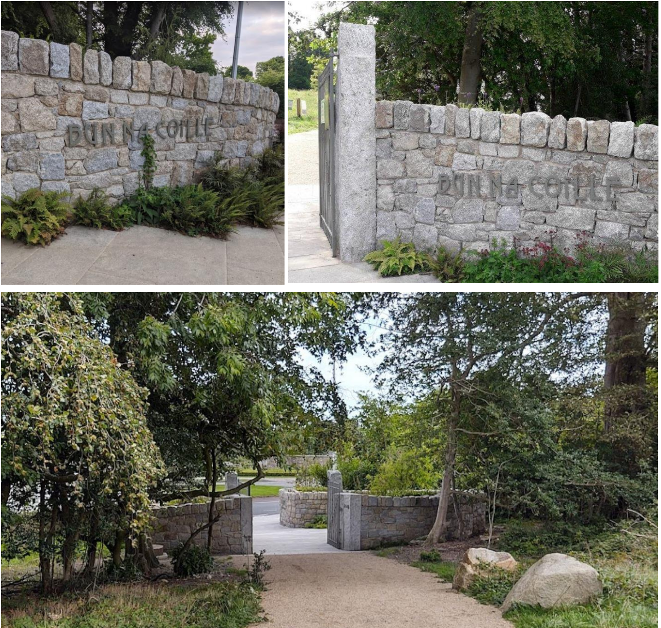
Figure 14-16: Reference images of Fern Hill Gardens, Dublin 18, illustrating natural stone cladding on walls at the gated entrance of the park.
