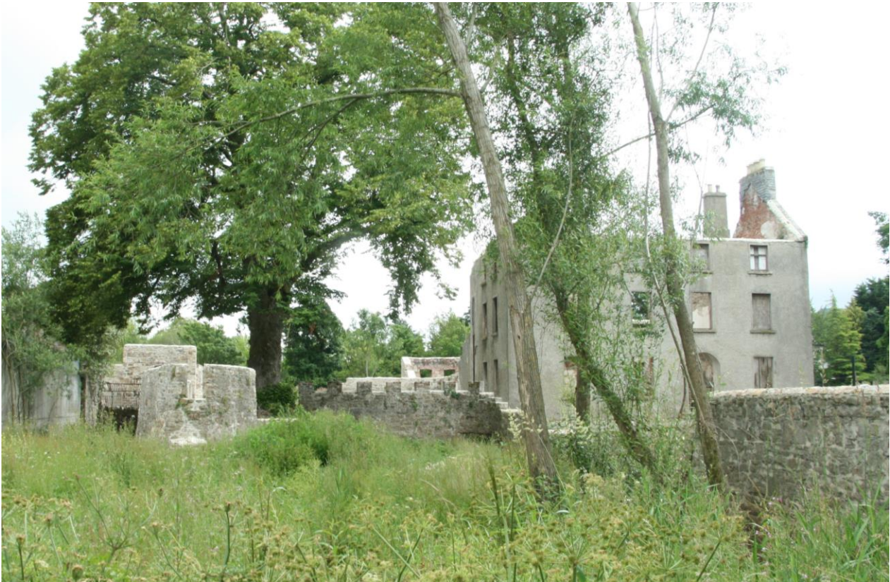
Figure 1: View from the west looking across the former headrace, with evidence of emerging vegetation. Suir Island House is on the RHS in the background. A large lime ( Tilia x europea ) tree is visible to the left of the house.
