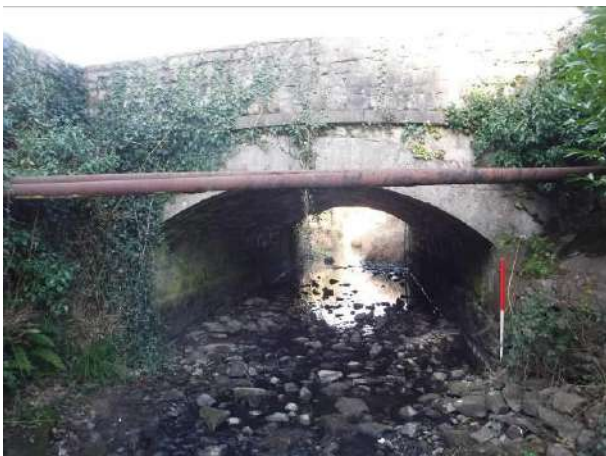
Plate 23 Small Bridge, facing north
