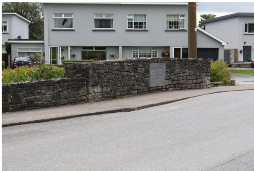
Plate 11: Upstream parapet of Small Bridge, seen from the road side
