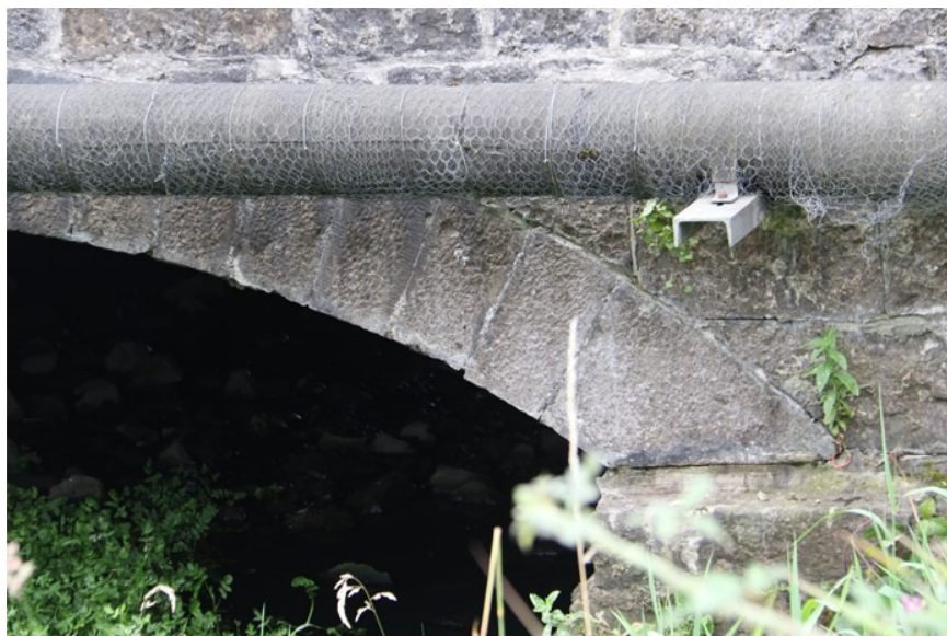
Plate 3: Detail of arch ring on upstream side of bridge
