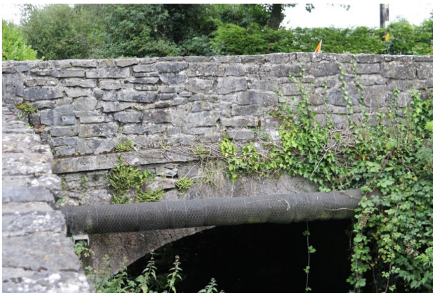
Plate 12: Upstream face and parapet of bridge
