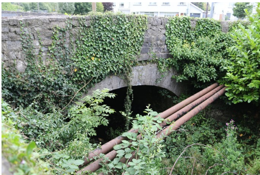
Plate 10: Downstream side of Small Bridge
