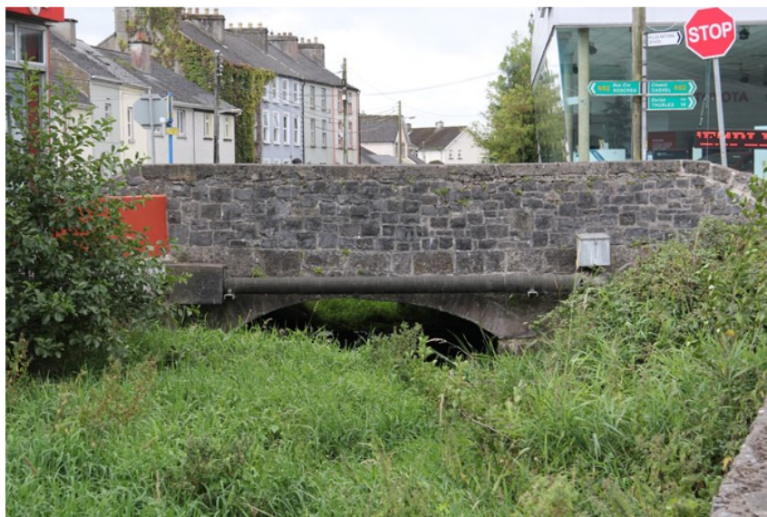
Plate 1: Upstream face of O'Dwyer Bridge
