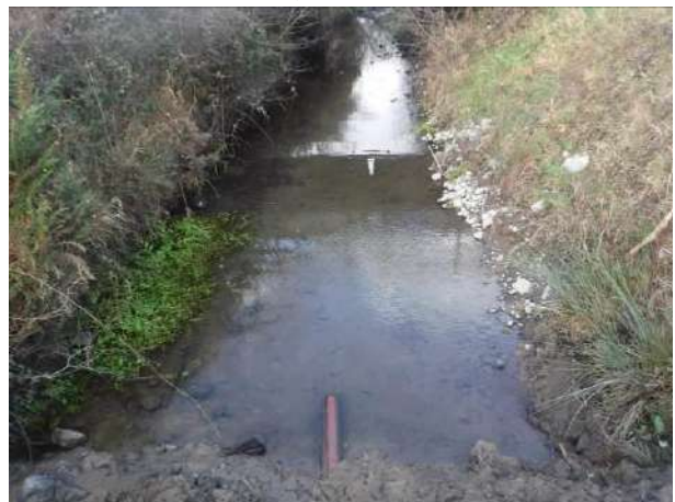
Plate 28 Southern Area Section 3, facing north
