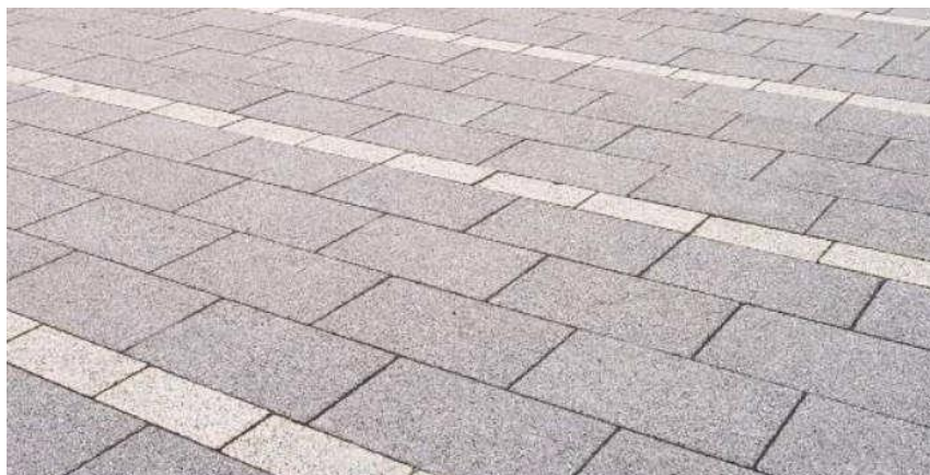
Figure 2-1 Surface Finish – Secondary Pedestrian areas
