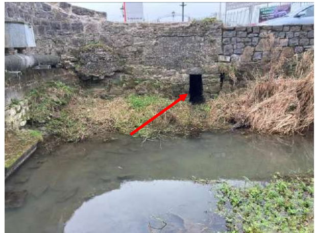
Plate 12 Drainage outlet upstream of O'Dwyer's Bridge, facing west
