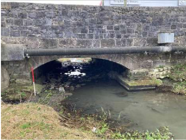
Plate 13 O'Dwyer's Bridge, facing south
