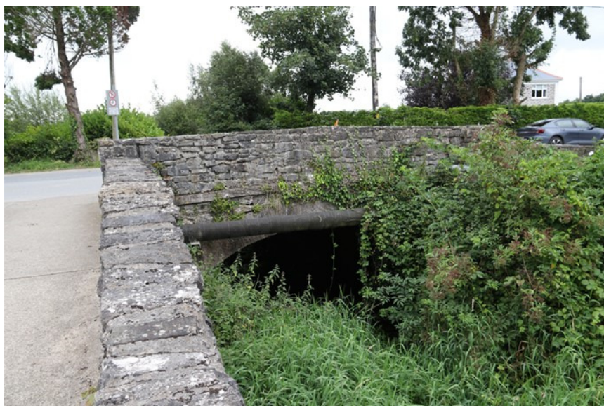
Plate 9: Upstream side of Small Bridge
