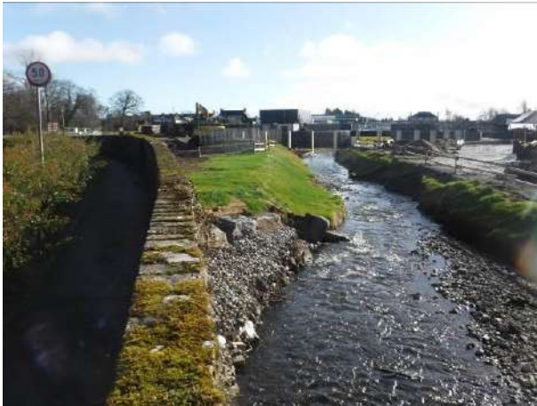
Plate 1 New channel upstream, facing south
