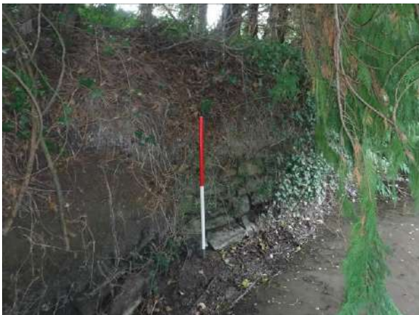
Plate 17 Earthen bank with possible façade walling, facing northwest
