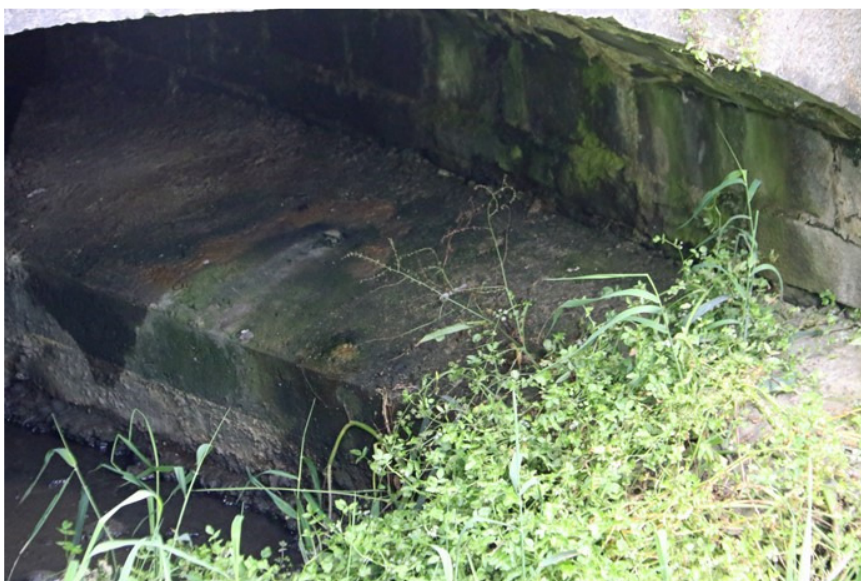
Plate 4: Shelf beneath the bridge
