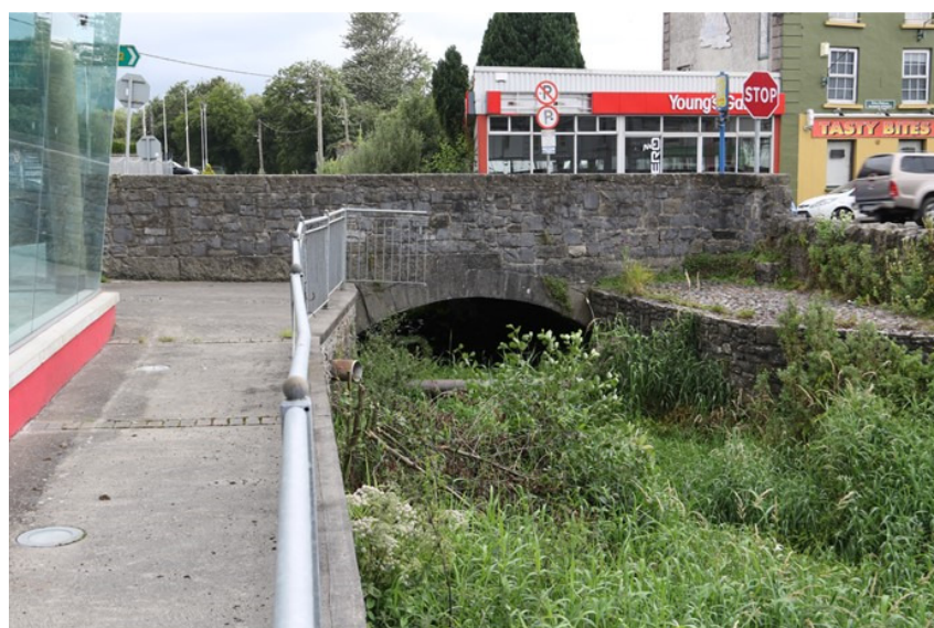
Plate 2: Downstream face of O'Dwyer Bridge
