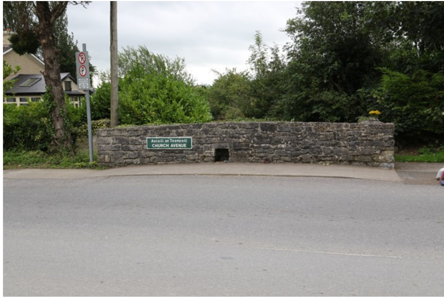
Plate 13: Downstream parapet of Small Bridge
