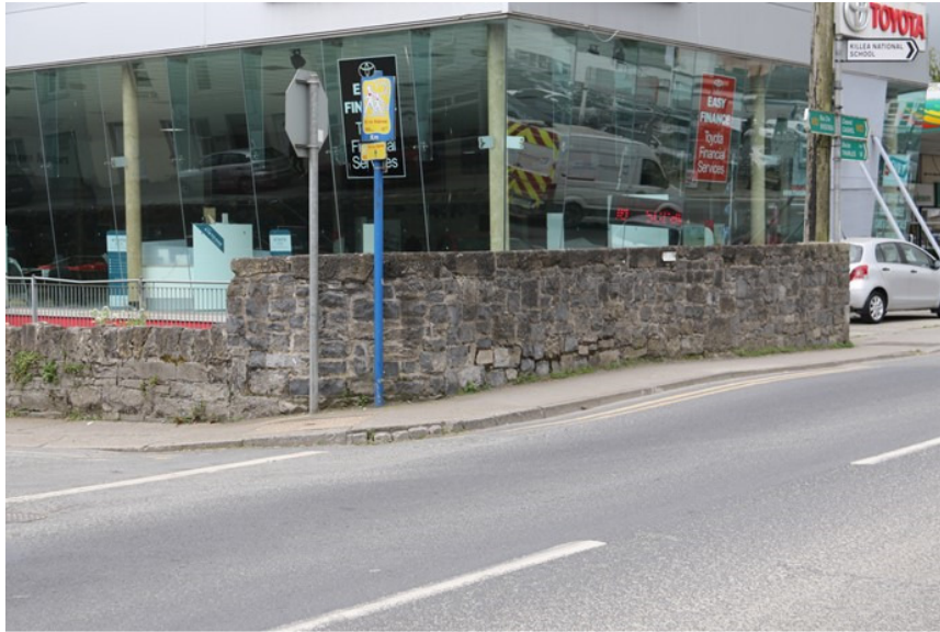
Plate 7: Downstream parapet on side facing the road
