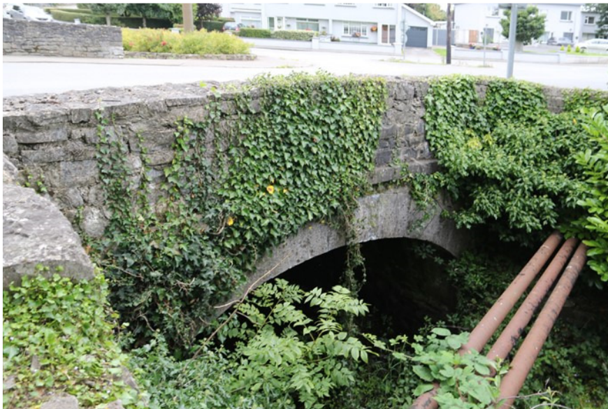
Plate 14: Downstream face and parapet
