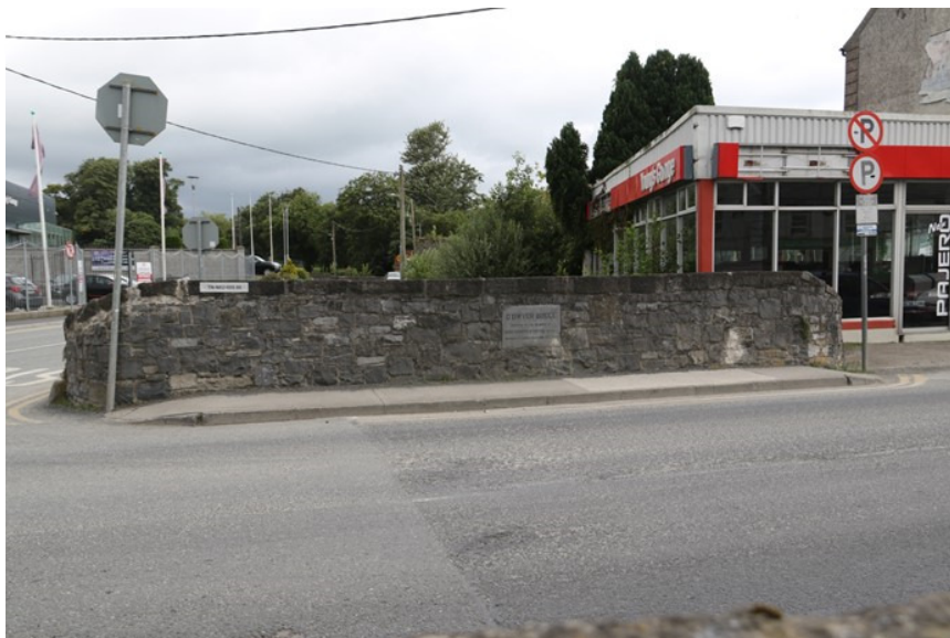
Plate 5: Upstream parapet on side facing the road
