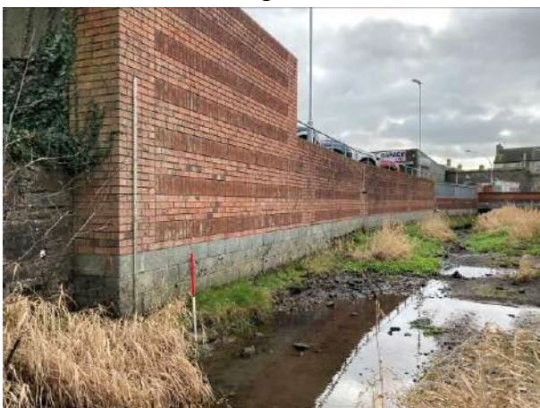
Plate 5 Modern Wall bounding river at Young's Garage, facing southeast
