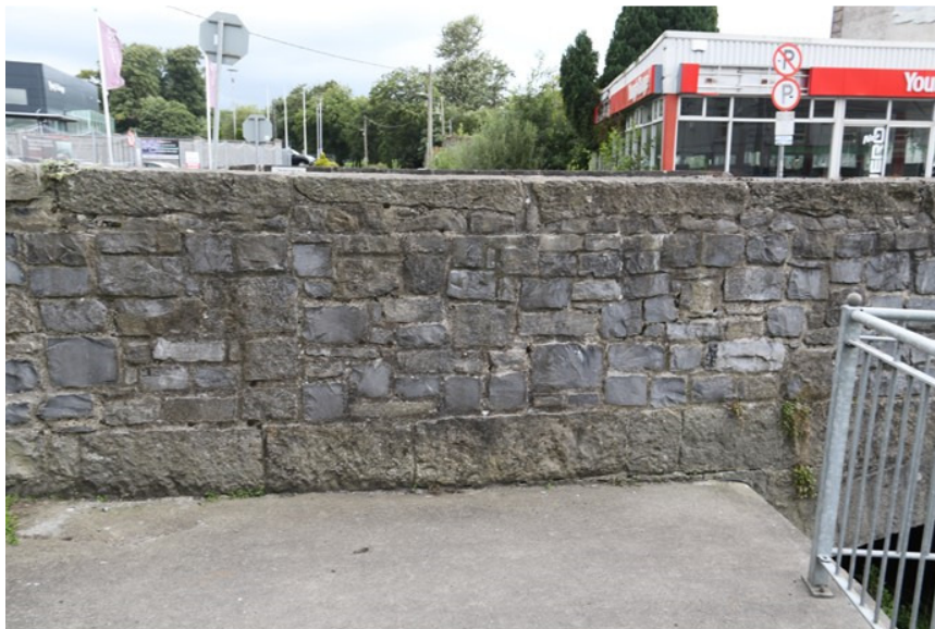
Plate 8: Detail of rear of downstream parapet
