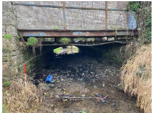
Plate 10 Timber and steel decked access bridge, facing north
