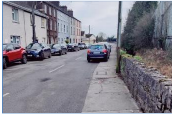
Figure 6-9 Blocked Footways by parked vehicles
