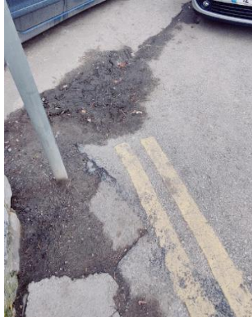
Figure 8-11 Area of Water Ponding on the East of the N62 / Blackcastle Road Junction
