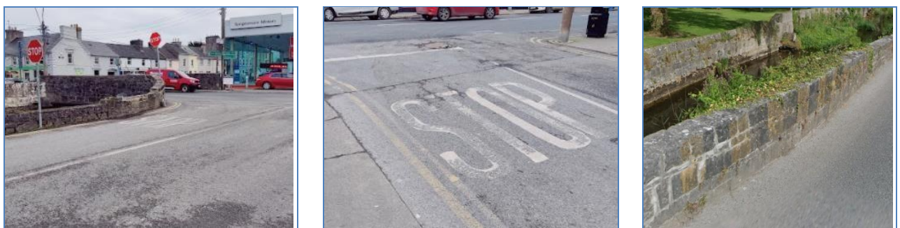
Figure 5-5 Faded Road Markings at the N62 / Blackcastle Road / The Mall Junction and Blackcastle Road
