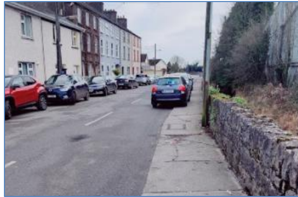
Figure 26-5 Blocked Footways by parked vehicles
