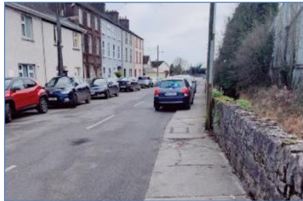
Figure 3-5 Blocked Footways by parked vehicles
