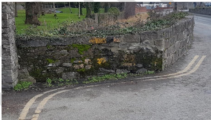
Figure 2-2 Road Markings at Town Park Entrance Boundary Wall
