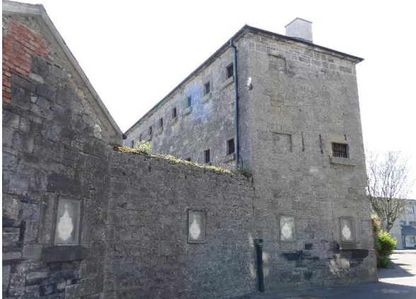
Fig. 104: The north gable of the gaol cell block. A walkway originally connected the block and governor's house at the upper level.
