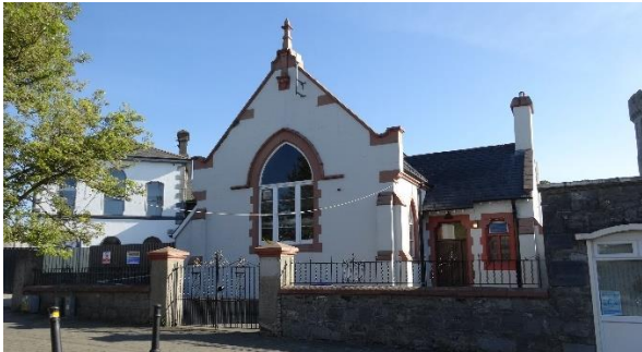
Fig. 40: Historic railings, gate and stone boundary wall enclose the tourist office in Banba Square.
