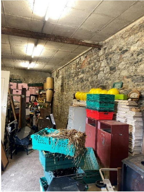
Fig. 160: Rear wall of Castle Shed viewed from the inside, note mix of historic masonry.
