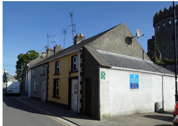
Fig. 31: Typical painted render finish to on O'Rahilly Street with a two-tone colour scheme using a contrasting colour to define features and openings. Pitched roofs covered with slates and clay chimney pots.
