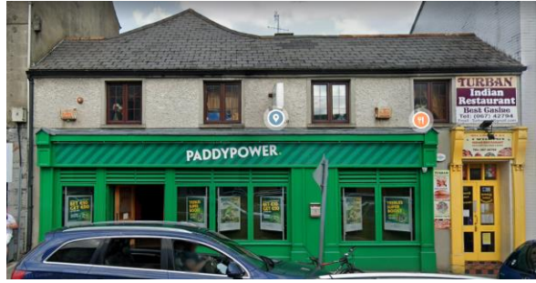
Fig. 37: Well-preserved traditional timber shop front, Kickham Street. The monotone colour scheme and branding and additional signage however, detracts from the historical features. The property has numerous modern interventions which has eroded its character above street level.
