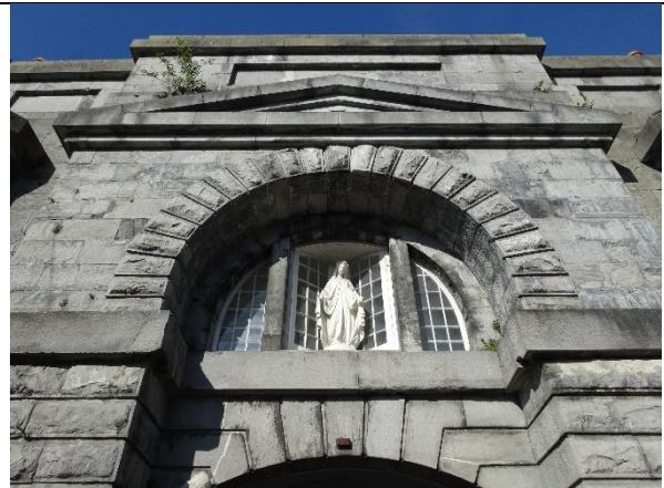
Fig. 131: The Diocletian window above the entrance gate. Condemned prisoners were hanged from this opening during public executions.
