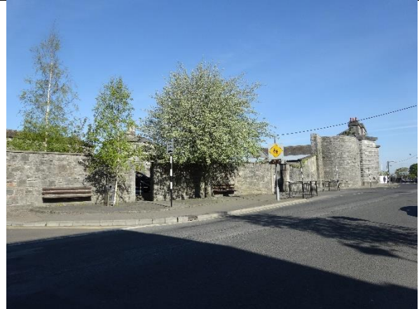
Fig. 105: Boundary walls of the former gaol viewed from the street.
