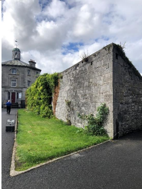
Fig. 148: View along north side flank wall.
