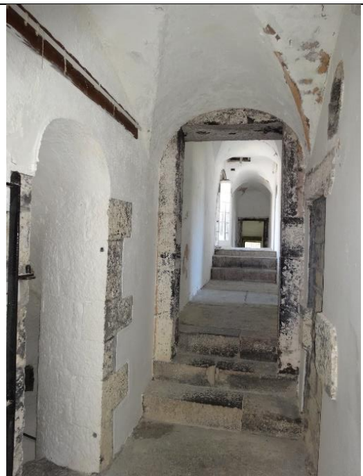
Fig. 139: First floor corridor leading to cells.
