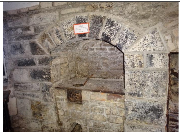
Fig. 73: Hotplate in segmental-arched niche.
