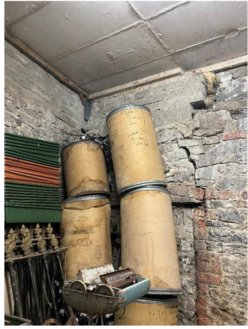
Fig. 161: Northwest corner of castle shed walls from the inside, note red brick opening reveal.
