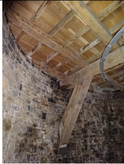
Fig. 168: Timber support below down stand beams, joists and floorboards.
