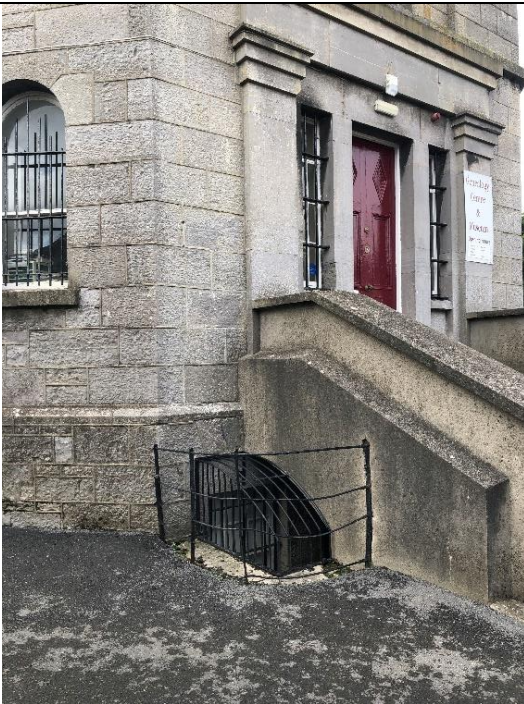
Fig. 64: View of basement access below main entrance stair
