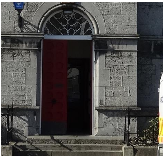
Fig. 34: A fine example of a historic timber door with brass features and decorative fan light above of the Garda station is a positive asset to Banba square streetscape.
