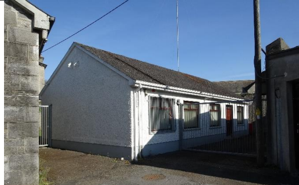
Fig. 123: Later 20 th century office building within yard [Note: white rendered Building 2 proposed for demolition]
