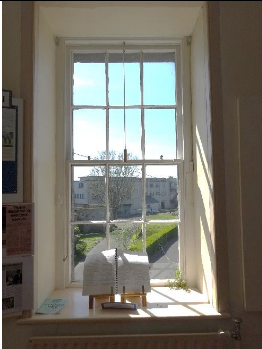
Fig. 86: Six-over-six timber sash window.
