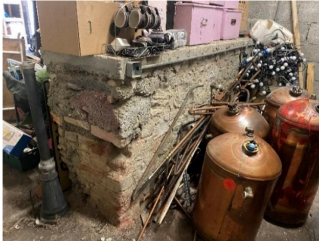
Fig. 164: Low section of masonry walling located within the castle shed.
