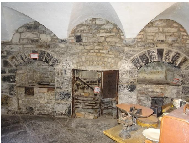
Fig. 72: Former kitchen in basement with vaulted ceiling.
