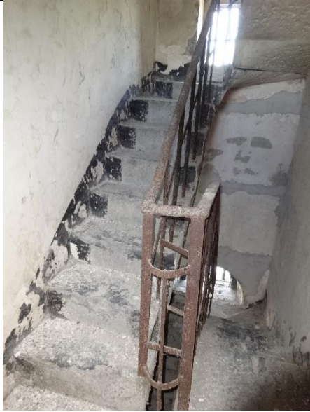
Fig. 113: Cantilevered stone stairs with wrought-iron balusters and handrails.
