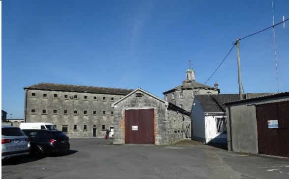
Fig. 122: The second cell block was modified for use as a store. Its upper floors were removed, and it received a new roof and gable-end doors.
