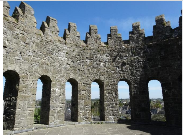
Fig. 157: The castellated parapet with arcade of window openings at the top of the tower.
