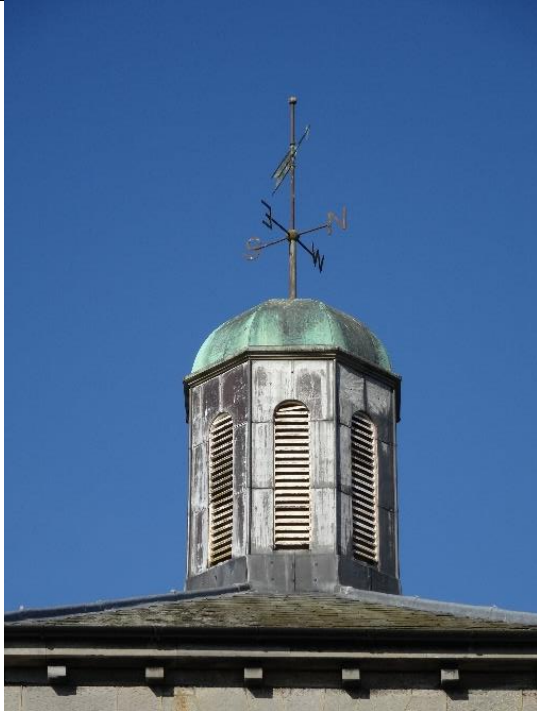
Fig. 62: Copper-domed cupola to apex of octagonal roof.
