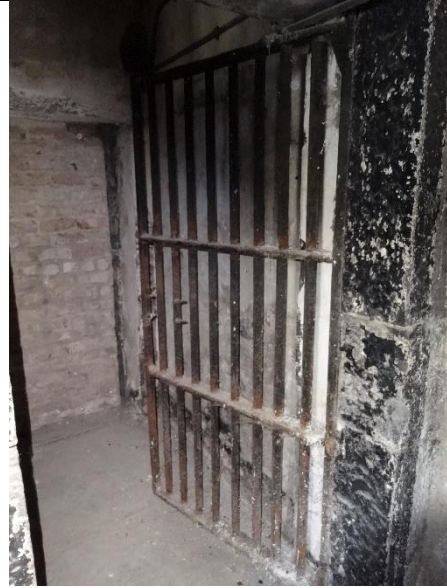
Fig. 114: Wrought-iron gate.
