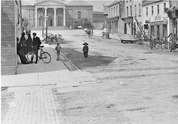
Fig. 44: Kickham Street looking towards Banba square from Castle street shows the historic cobbled crossing points and gullies, dirt roads and flag stone pavements. Robert French (Lawrence Collection), Peter Street, 1865-1914. L_ROY_09654
