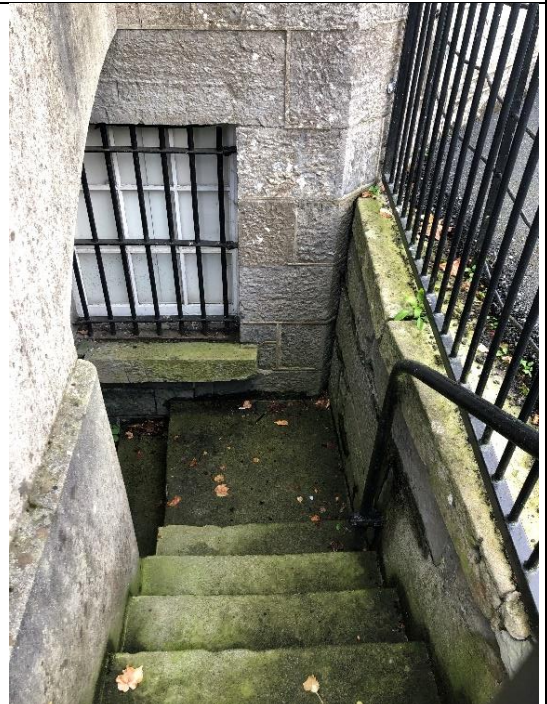
Fig. 65: Staircase to basement level entrance.
