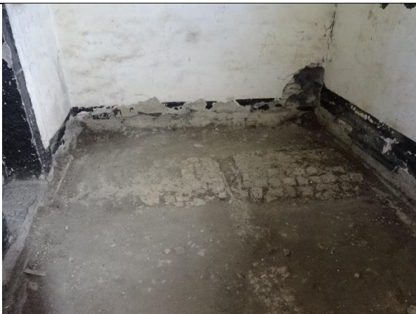
Fig. 117: Upper side of the vaulted ceiling, visible following removal of floorboards.
