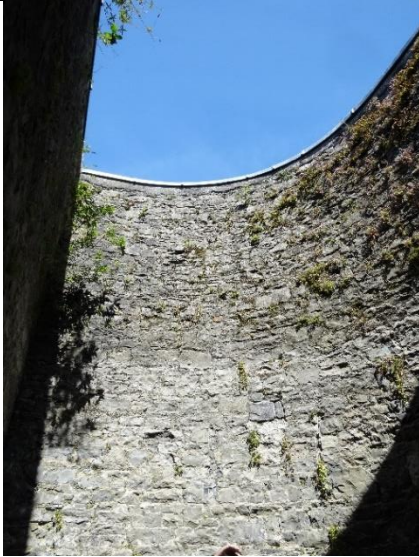
Fig. 142: High, curving wall of a prison yard from inside.
