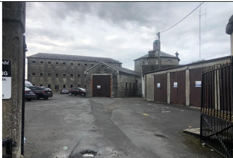
Fig. 121: View looking towards single storey cell block with modern shed structure visible to the right of the image.
