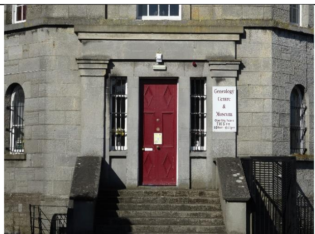
Fig. 61: Ashlar doorcase with pilasters and entablature, barred sidelights. Diamond and rectangular flat panels to painted timber door.
