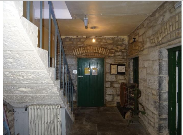
Fig. 71: Hallway in basement.
