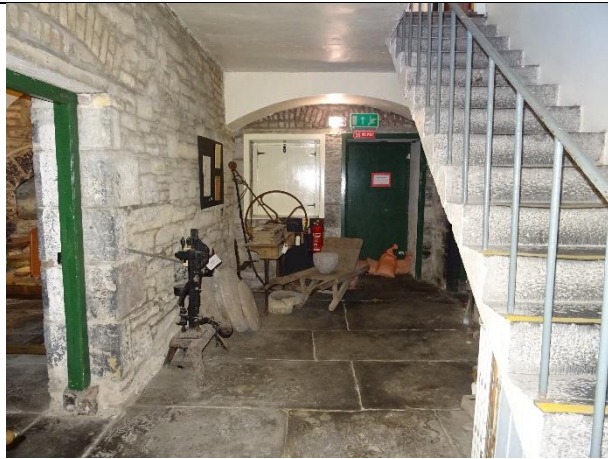
Fig. 70: Cantilevered stone staircase rising from basement to entrance hall.
