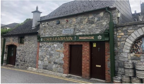
Fig. 36: Traditional style timber signage with appropriate style of lettering to pub on O’Rahilly Street.
