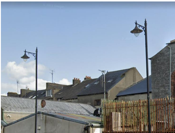
Fig. 50: Decorative street lamps to car park on O'Rahilly Street are a positive contribution. 2021 © Google Streetview.
