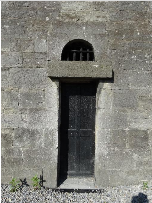
Fig. 108: Narrow entrance door with round-arched vent to cell block.
