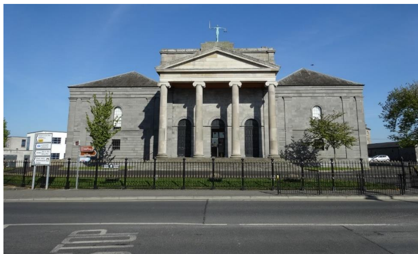
Fig. 43: The courthouse 2021. Railings to the south of the courthouse are intact except the gate posts and gates to the west have been repositioned and the lanterns have been removed. The paving to the base of the railings is modern with concrete kerbs and asphalt road surface.
