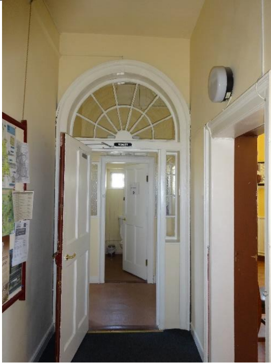
Fig. 84: Round-arched door opening with fanlight.
