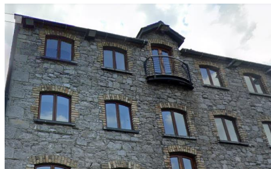
Fig. 39: While the finish likely would have been lime plaster, the exposed stone with brick surrounds offers a please texture and tones to the townscape.
