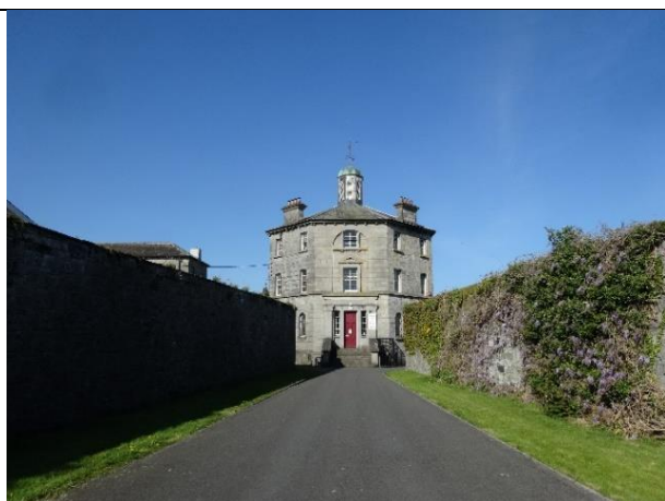
Fig. 60: The octagonal governor's house at the centre of the former gaol complex. Avenue from gatehouse to governor's house is bounded by tall random-coursed stone walls.
