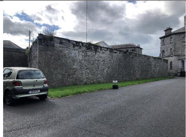
Fig. 145: Limestone wall to front of governor's house, south side flank wall.
