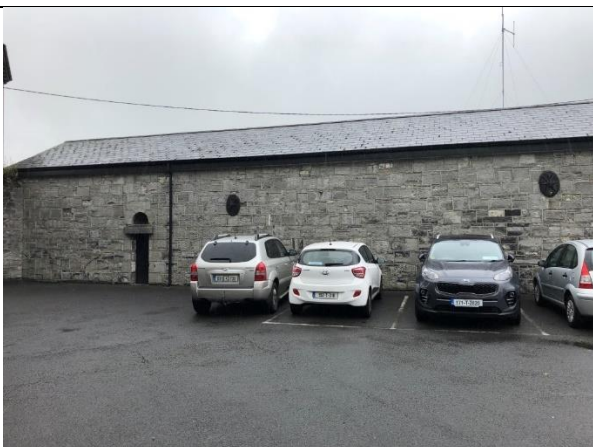
Fig. 126: View of single storey cell block from the west.
