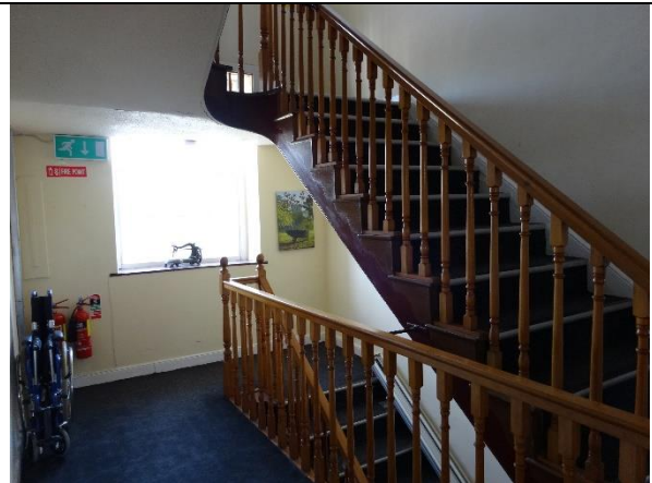
Fig. 91: Replacement balusters, handrails and newels to timber dog-leg stairs.
