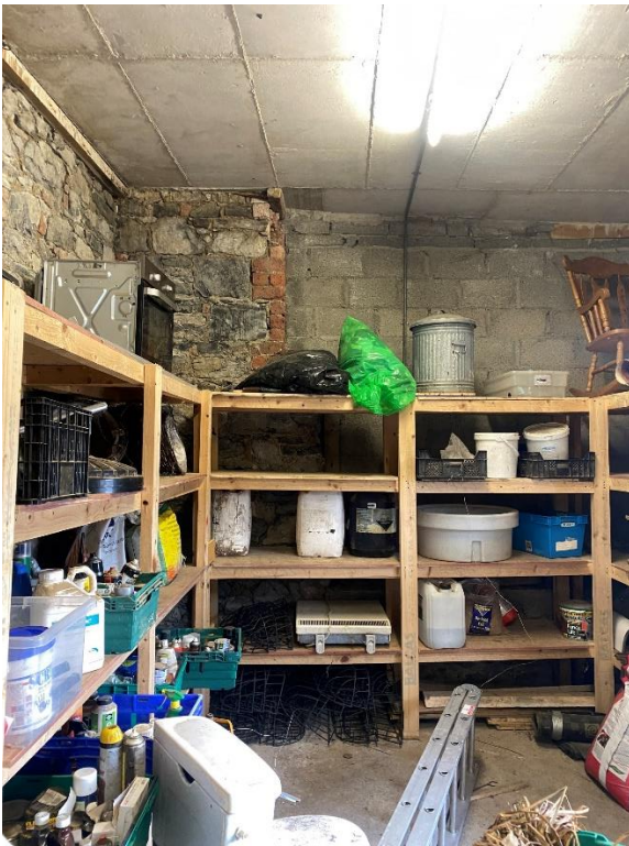
Fig. 160: Rear wall of Castle Shed viewed from the inside, note mix of historic masonry.
