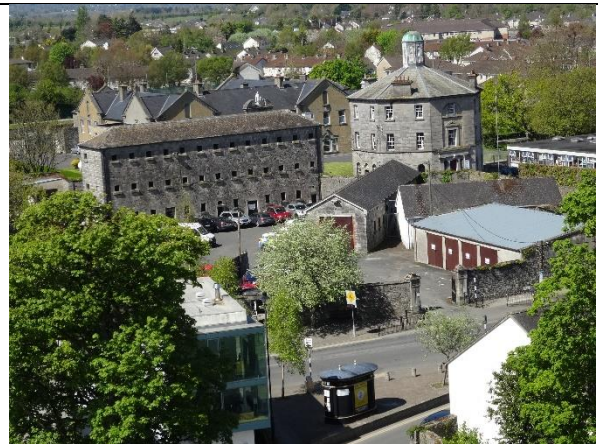
Fig. 107: A view of the former gaol from the top of Nenagh Castle.
