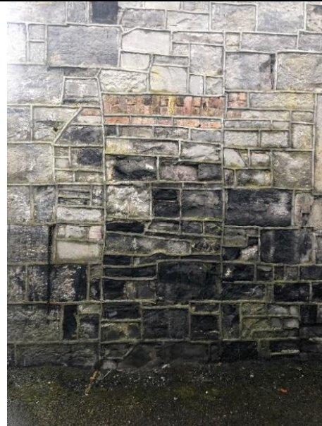
Fig. 125: Cementitious strap pointing and blocked up opening
