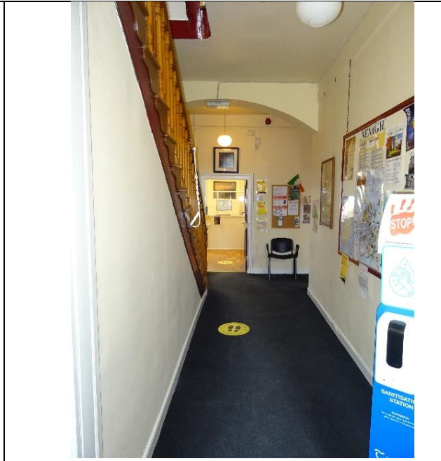
Fig. 81: Principal staircase with modern replacement balusters, newels and handrail.
