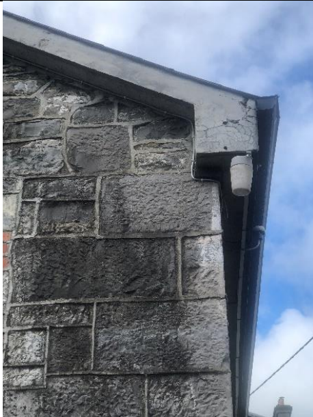
Fig. 124: View of concrete barge cast onto existing building
