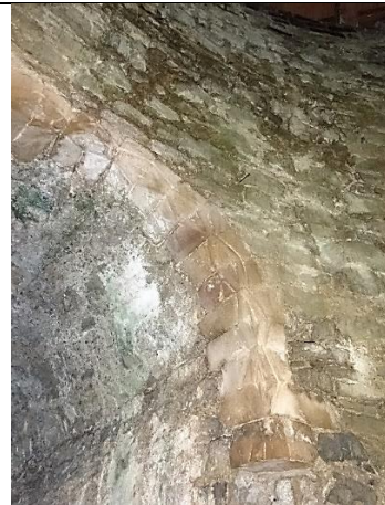
Fig. 172: Doorway with shouldered arch.
