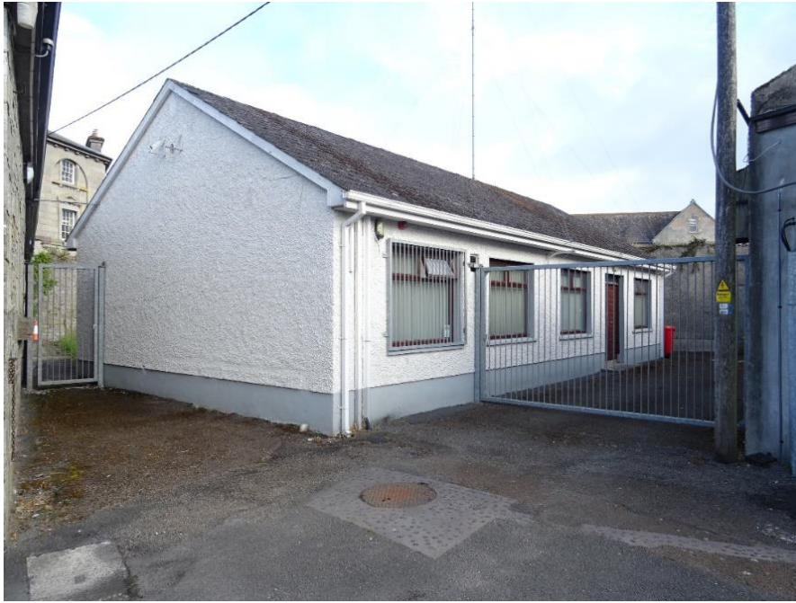
Fig.5: Bungalow building within the gaol complex proposed for demolition.
