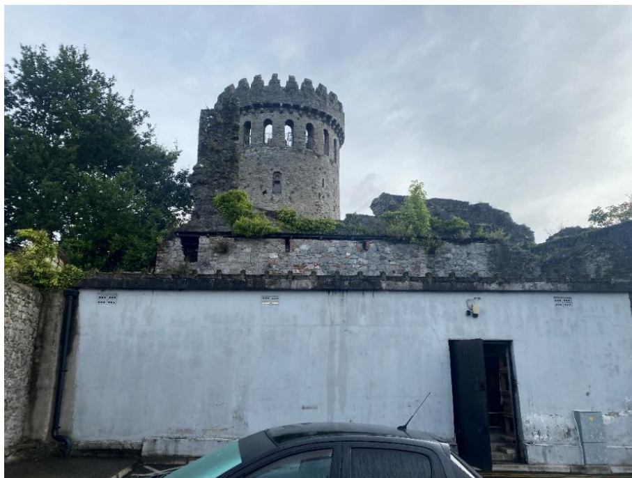
Fig.4: 'Castle Shed' Building proposed for demolition.
