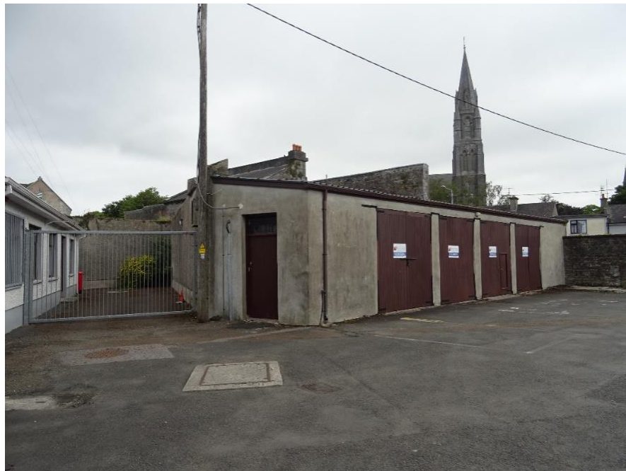
Fig.6: Garage building within the gaol complex proposed for demolition.
