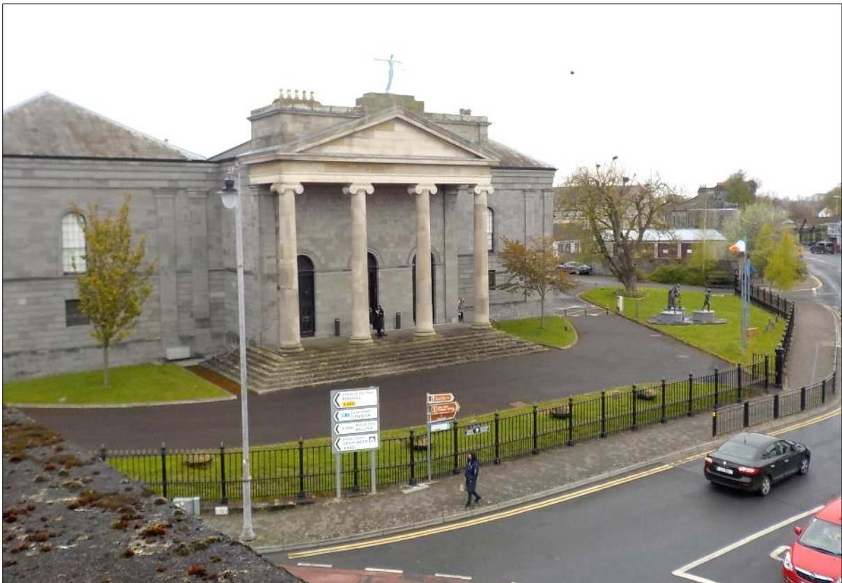
Plate 10: View of the southeast facing façade of Nenagh Courthouse and the north-western portion of Banba Square
