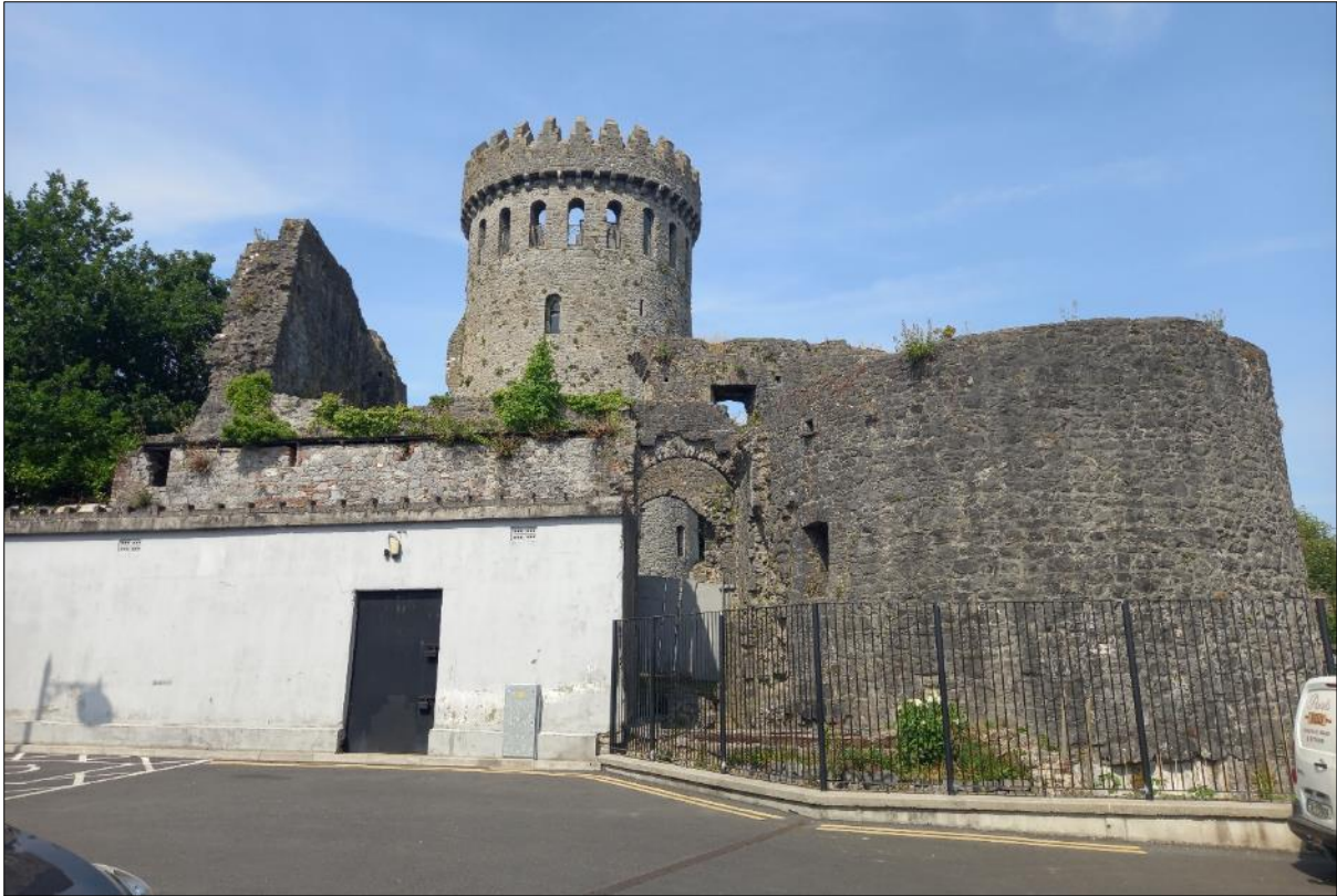
Plate 5: Exterior view of the gatehouse of Nenagh Castle as viewed from the O'Rahilly Street carpark. Modern lean-to structure occupies the location of the original western flanking tower of the gatehouse, the modern structure is proposed to be demolished as part of the NHCQ project
