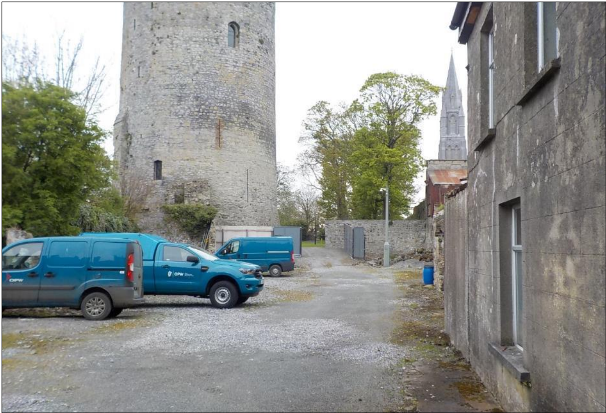
Plate 9: View of the existing OPW yard located to the east and southeast of the keep of Nenagh Castle
