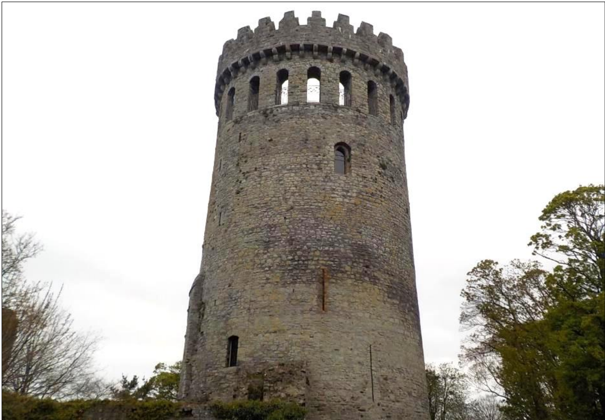
Plate 3: View of the eastern elevation of the circular keep of Nenagh Castle as viewed from the existing OPW yard, portion of curtain wall evident in foreground
