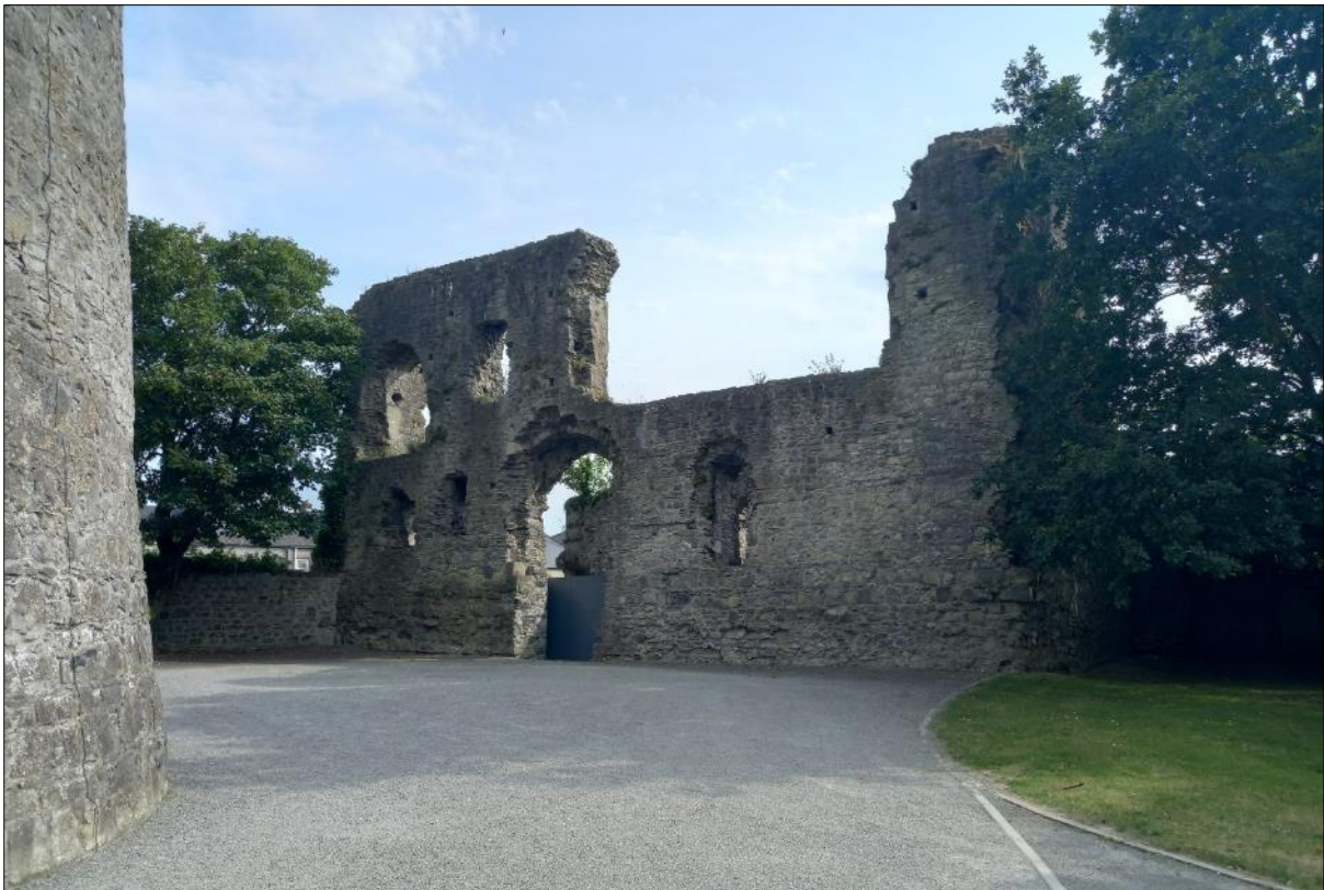
Plate 6: View of the gatehouse hall as viewed from the base of the circular keep of Nenagh Castle, facing south
