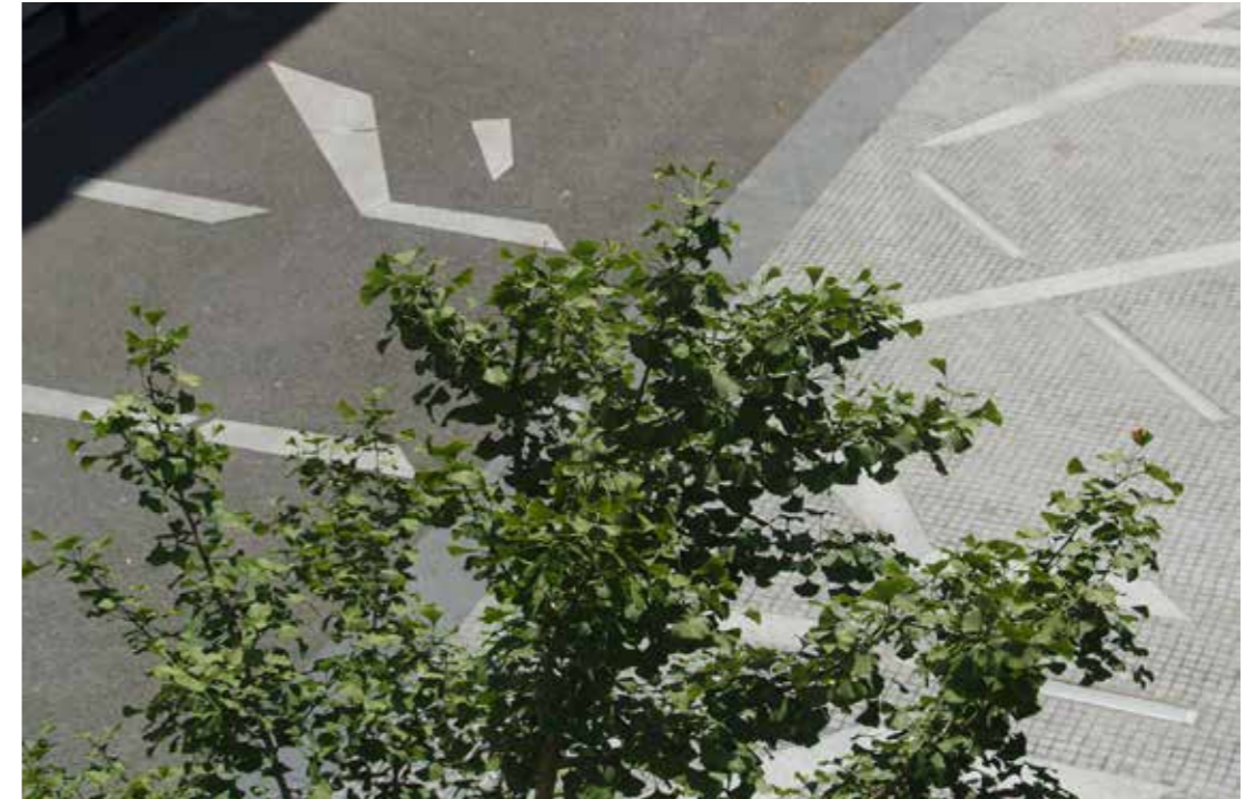
Embedments in the surface instead of paint
