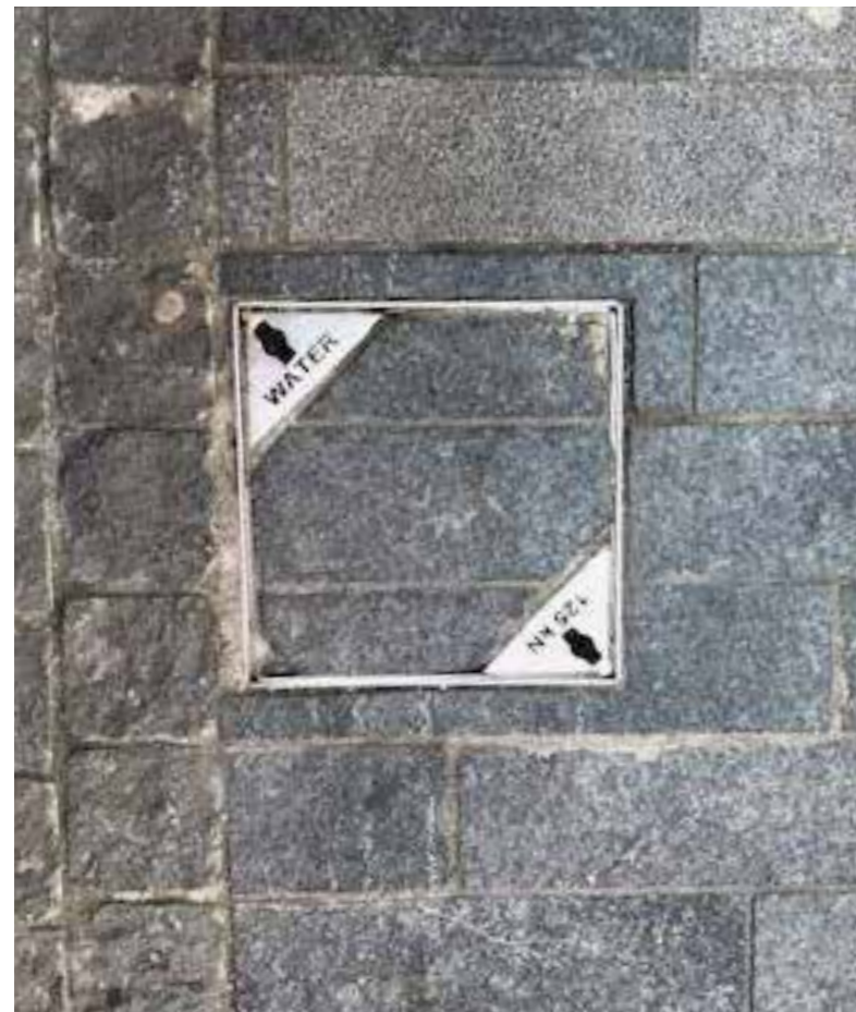
Services integrated with paving pattern
