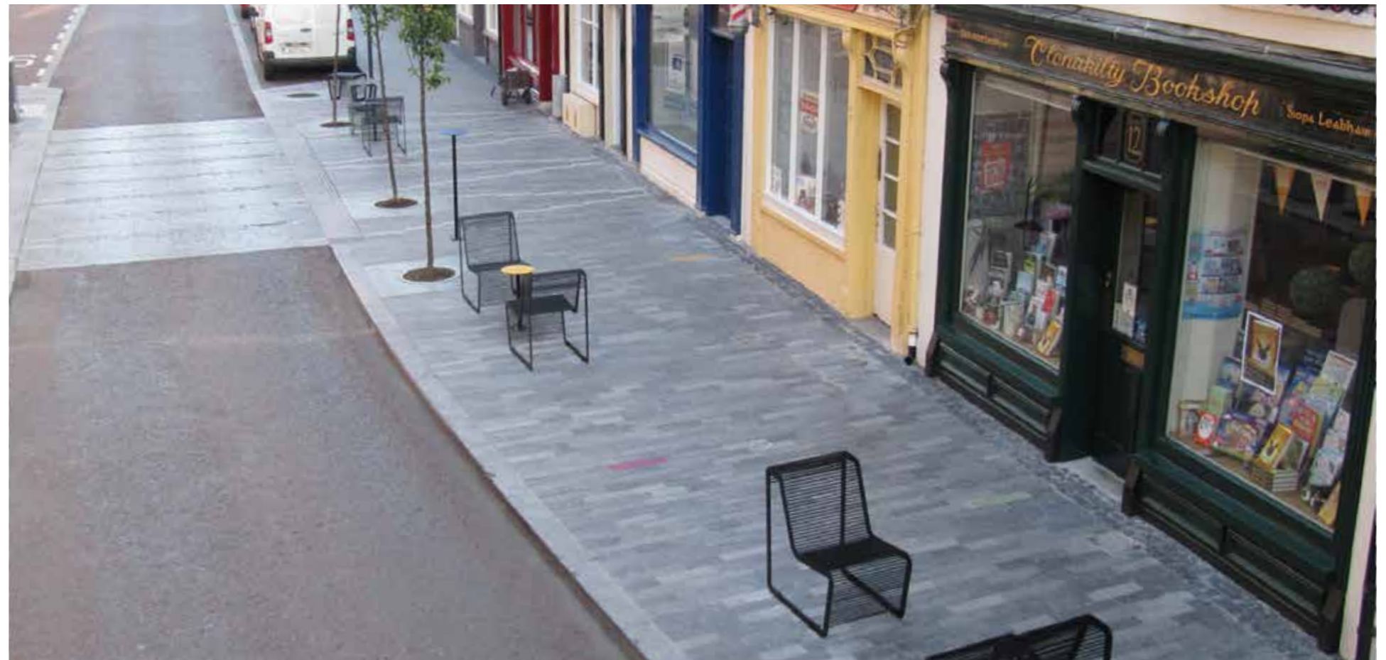
Upgraded footway with natural stone (Limestone) in Clonakilty, Co. Cork.
