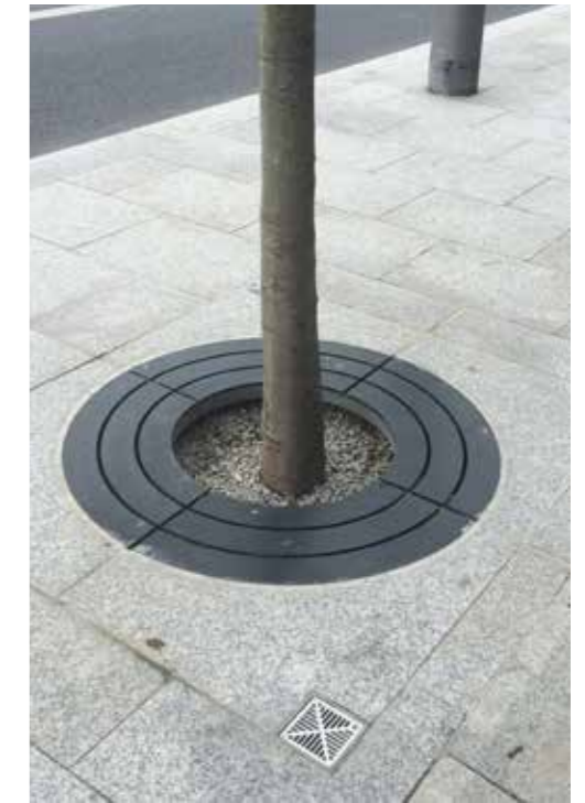
Tree grille and aeration vent
